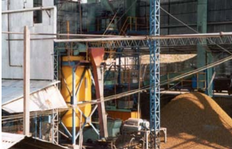
Palm oil production plant in Aguaytia, Peru: Peoples living conditions are improved
